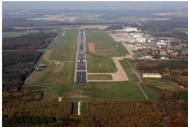
Upgrading Frankfurt-Hahn Airport Concrete/Asphalt surface approx. 65.500 m 2 , Runway extension, Taxiway- and Drainagesystems, Threshol 03, central retention basin (44.000 m 3 ) (© picture: PlanePictures.net, Reiner Bexten for Frankfurt-Hahn Airport)
